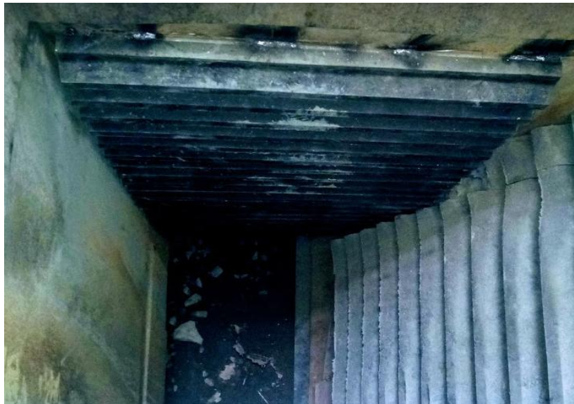
Figure 1 – Tooth plate VSS60-80 mm (Source: WP systems s.r.o.)
